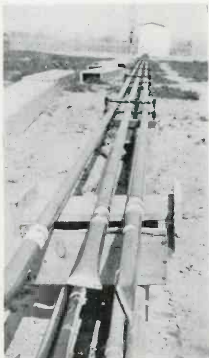
▼ Transmission line as sealed and tested daily during construction
