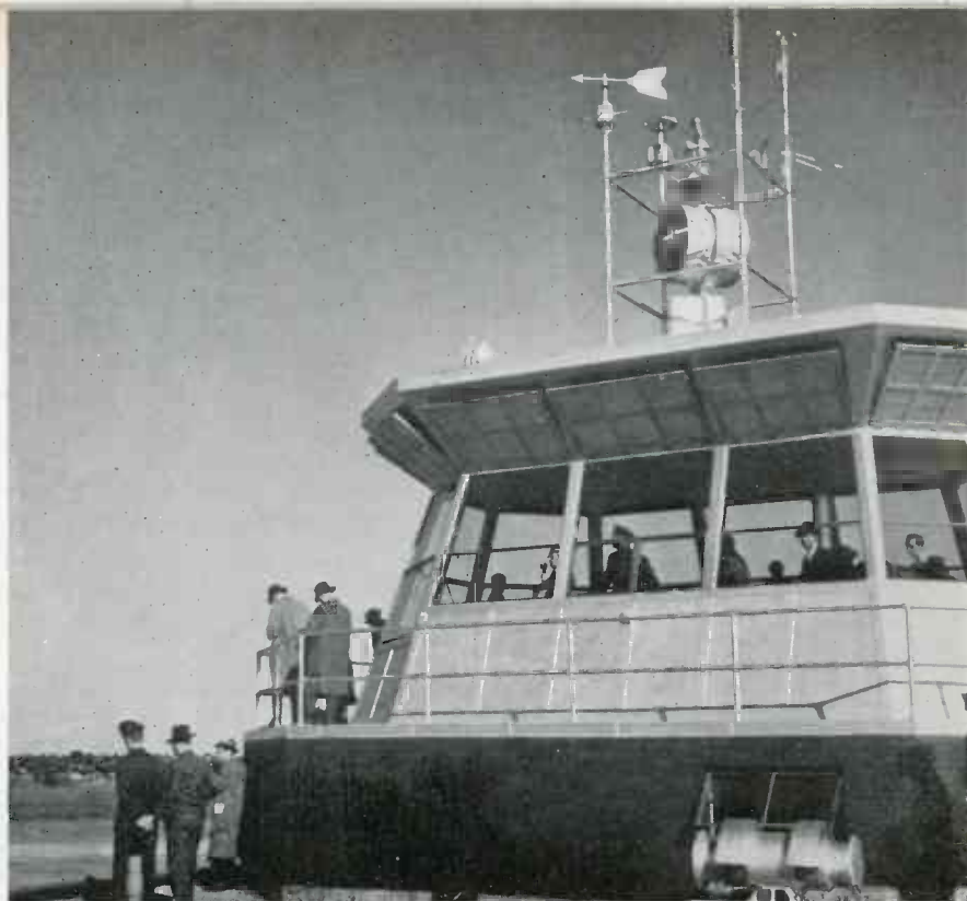
Tower for uhf landing and other electronic traffic controls at LaGuardia Field
